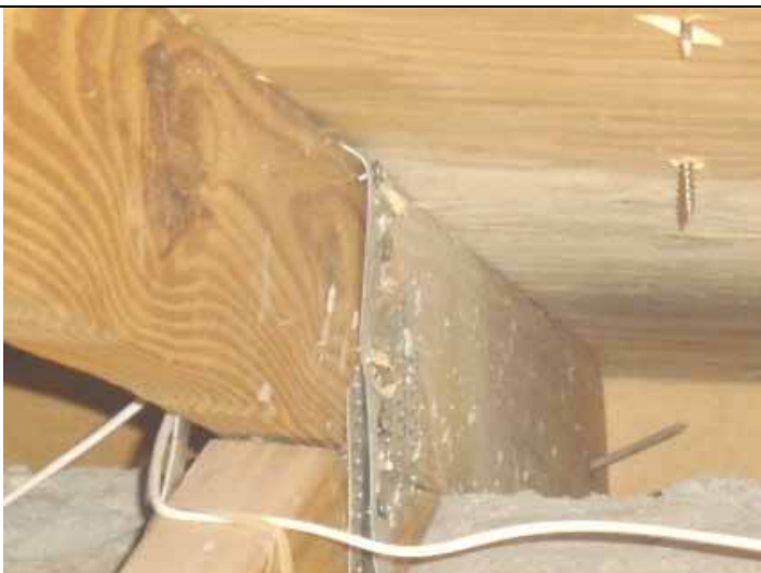
Roof to wall attachment
