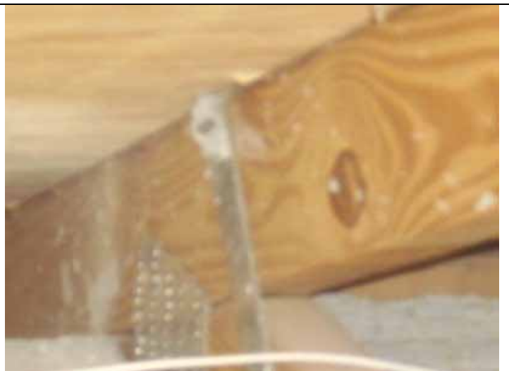
Roof to wall attachment
