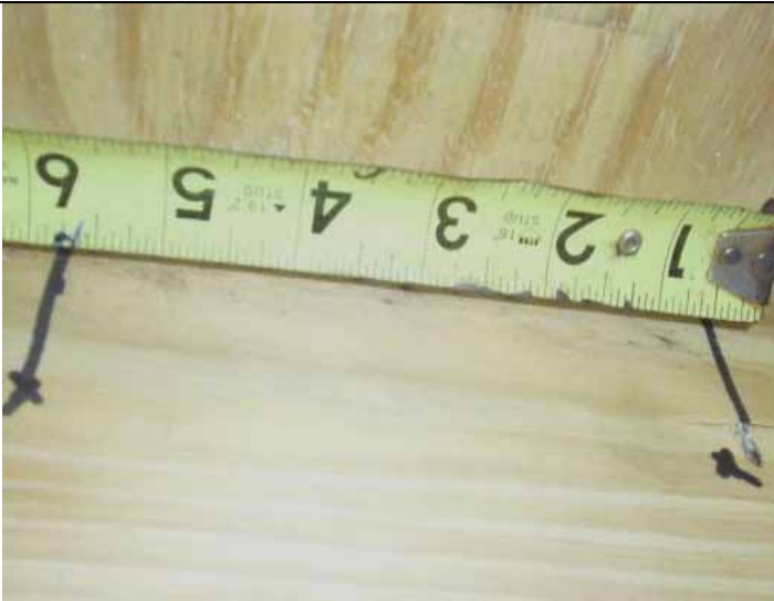
Roof deck attachment
